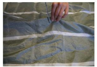
Illustration 3: Cut in upper Incomat<sup>®</sup> layer, with a length of 3 - 5cm
