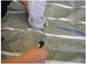
Illustration 10: Place hose over Incomat<sup>®</sup> ring and fixation of hose clip
