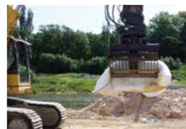
Installation with the aid of an excavator or similar
