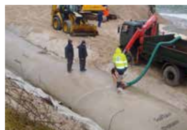
Filling the tubes (suction dredger, slurry pump)
