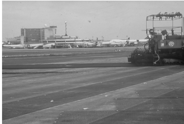
Figure 4. Installation of the polyester reinforcement at Brussel Airport in 1979
