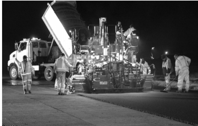
Figure 7. Laying asphalt over polyester asphalt reinforcement
