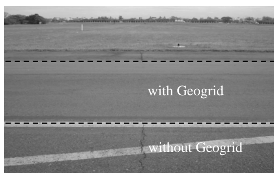
Figure 6. Joints of the concrete slabs reflect in the area where no reinforcement was used
