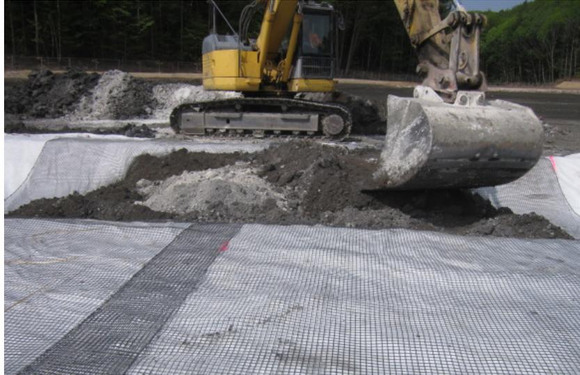
**Figure 6. Fixing geosynthetic in the anchor trench.**
