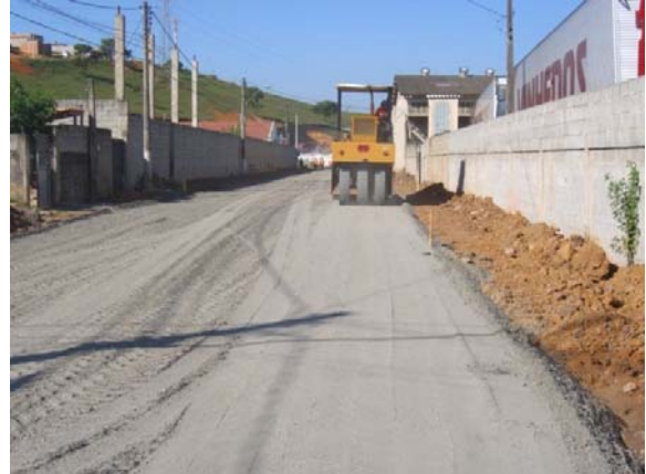
Figure 11. Compaction of base of BGS (graduated gravel).
