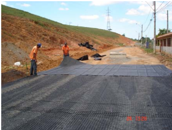
Figure 8. Installation of woven geotextile [GTW].
