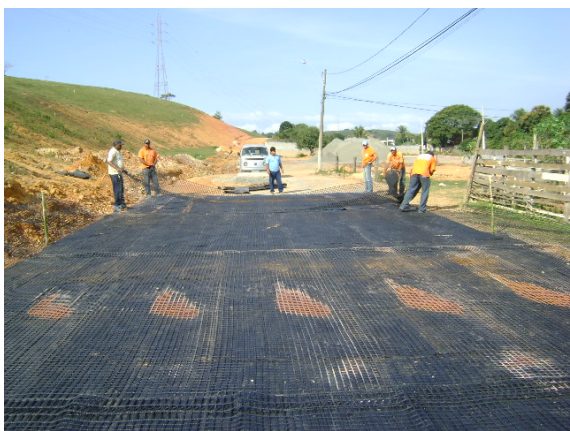
Figure 9. Installation of geogrid [GG] Fornit J600.
