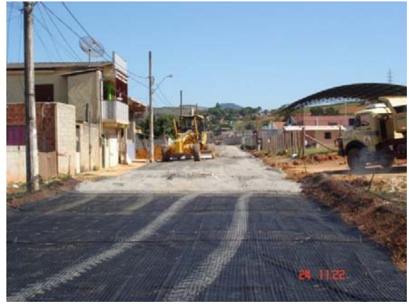
Figure 10. Construction base with BGS (graduated gravel).
