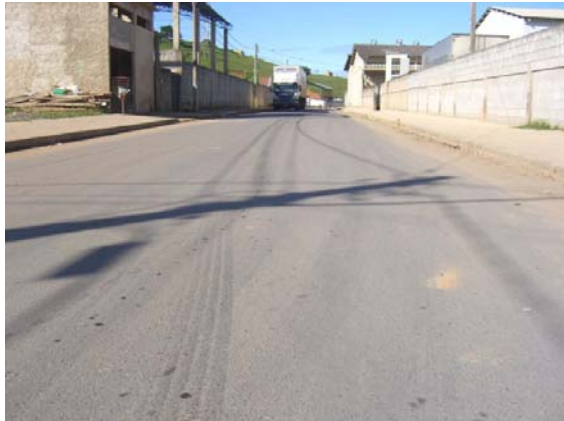
Figure 13. Pavement in operation and in perfect condition (December/2011).
