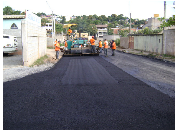
Figure 12. Constructio of asphalt concrete
