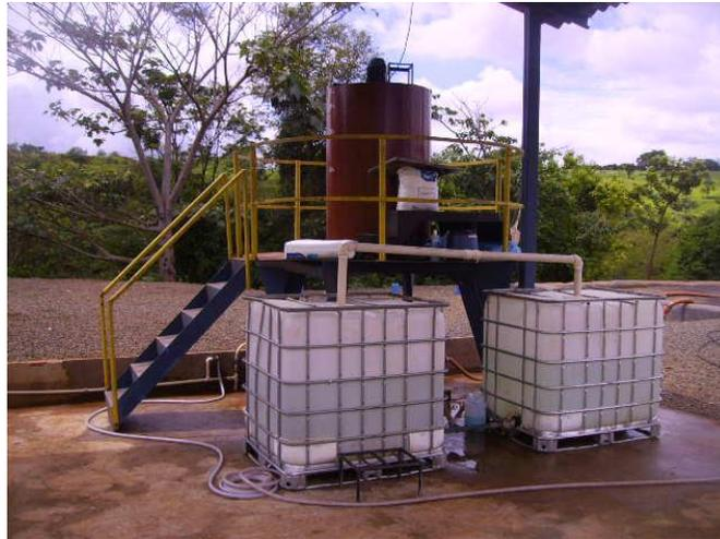
Figure 4. Polymeric Unit (responsible for the adequate dosage and addition of the flocculate solution into the effluents conduction)
