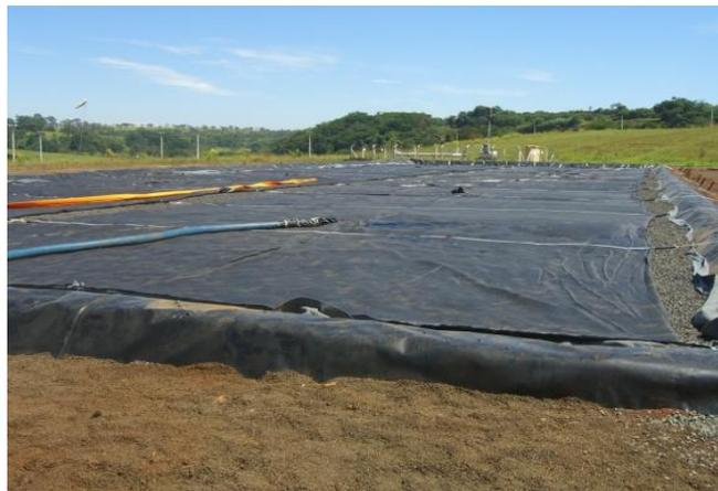
Figure 5. Drainage bed and geotextile tubes before filling
