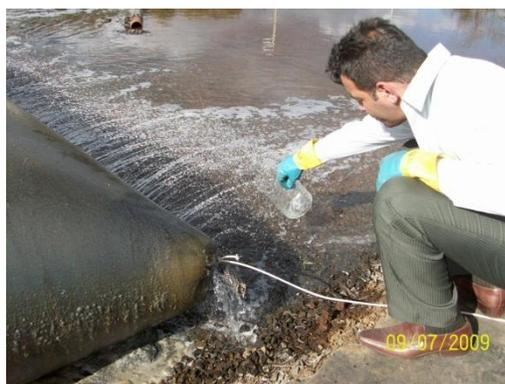
Figure 6. Geotextile tube during filling
