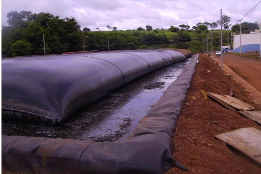
Figure 1. Geotextile tubes at Uberabinha wastewater treatment plant
