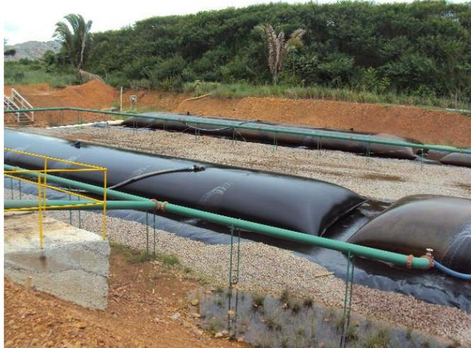
Figure 9. Geotextile tubes at hydroelectric power plant Santo Antônio
