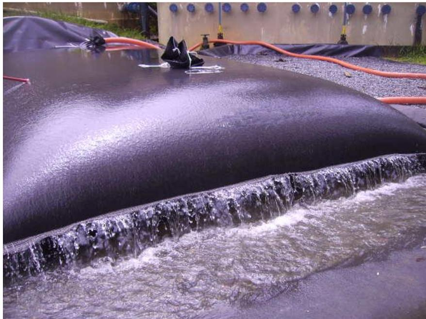
Figure 12. Filling of the geotextile tube
